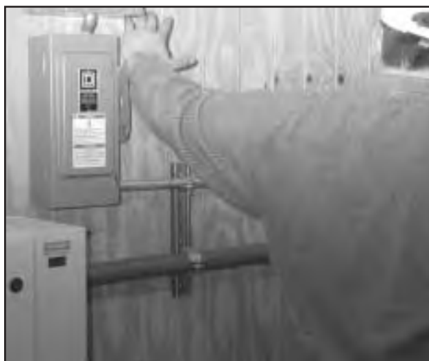
Figure 12-1. Proper method to safely bump or switch a disconnect lever on an electrical box.
