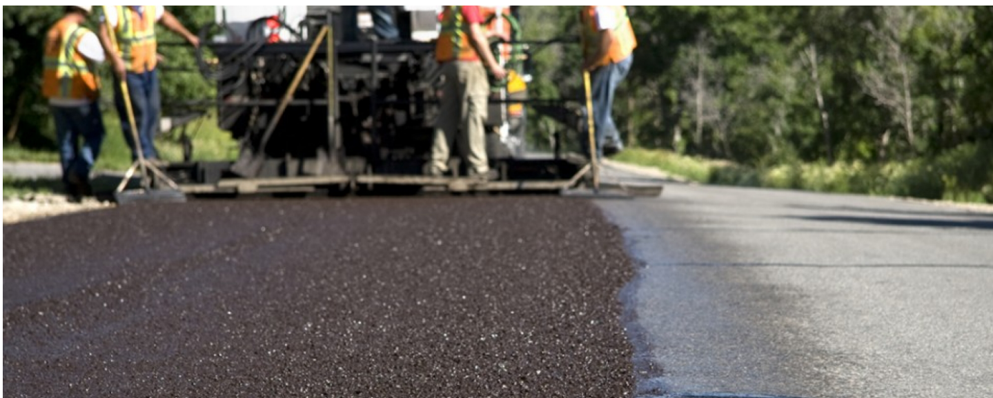
San Francisco Public Works crews install micro surfacing on an asphalt road. (San Francisco Public Works, 2020)
