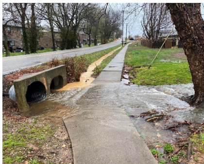
This picture displays muddy water coming from a development site just up the block during a rainfall event. Notice that the bigger stream is not as muddy as the water flowing in the stormwater drainage ditch. Sediment is the number one form of pollution to surface waters in Arkansas and across the United States.
