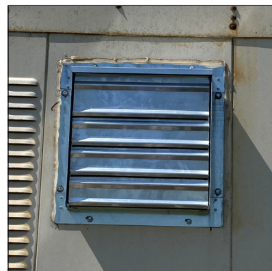
Figure 3. Exterior of the gable vent fan installed for the walk-in dehydrator (Clarksville, AR)
