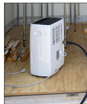
Figure 13. Placement of dehumidifier next to the door with drainage hose leading outside of the building (Clarksville, AR).
