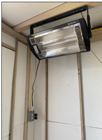
Figure 9. Ceiling mounted heater used in walk-in dehydrator (Clarksville, AR).
