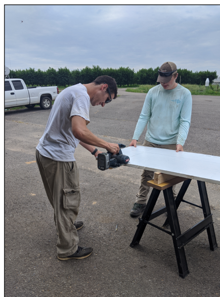
Figure 4. Fruit Research Station staff James McClellan (left) and Emory Johnson (right) cutting polystyrene foam board for insulation (Clarksville, AR).
