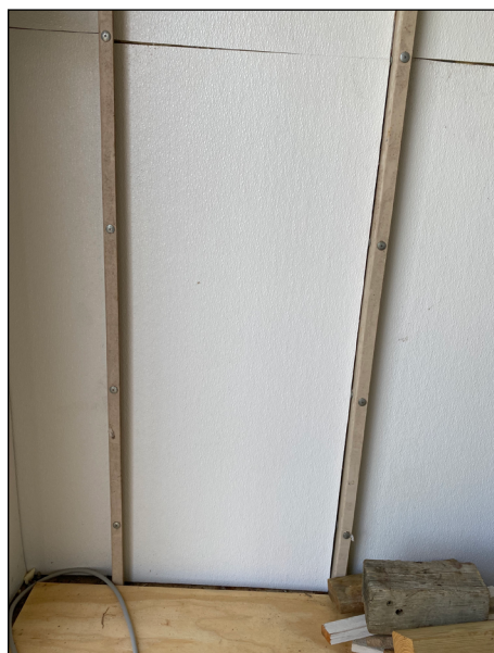
Figure 5. Insulation layers of fiberglass reinforced plastic (FRP) over polystyrene foam board in the walk-in dehydrator (Clarksville, AR).
