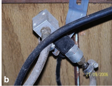
FIGURE 10. A solenoid valve (cube in b.) and oxygen tank can be a useful combination for oxygen backup. The solenoid valve is plugged into an electric receptacle (a.) which keeps the valve closed. In the event of a power outage, lack of electricity opens the valve and oxygen can flow to the fish. The tank should be well secured and all fittings in good condition to ensure oxygen does not leak from the system. Although this setup has a regulator, it does not include a flow meter, which is preferable.
