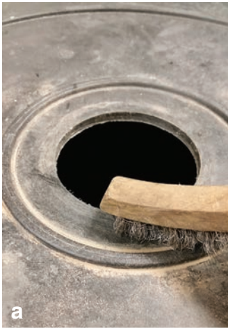
FIGURE 5. Use of epoxy putty to seal in a bulkhead fitting. 5a: Clean and rough up the area with a wire brush or sandpaper; 5b: cut off a portion of the epoxy putty; 5c: knead the putty together (always use gloves with this material) until the color is uniform; 5d: when the color is uniform roll into a ring and place around the bulkhead fitting; 5e: put the bulkhead fitting in place; 5f: tighten the fitting in place which will push the excess epoxy out; 5g: use the excess to form a wedge to help lock the wall and the fitting together. If there is not enough excess, prepare more putty and make a sufficient wedge.
