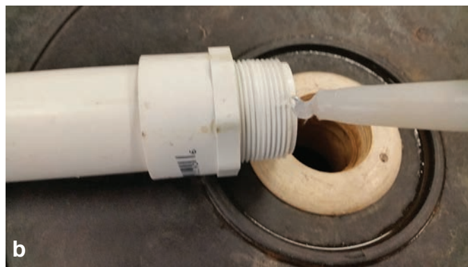
FIGURE 2. Sealing a leak between threads inside a bulkhead fitting. 2a: threads to be sealed; 2b and c: applying silicone sealant; 2d: threading complete, note the bead of silicone formed between the bulkhead and the pipe joint.
