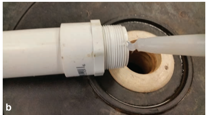
FIGURE 2. Sealing a leak between threads inside a bulkhead fitting. 2a: threads to be sealed; 2b and c: applying silicone sealant; 2d: threading complete, note the bead of silicone formed between the bulkhead and the pipe joint.
