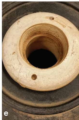
FIGURE 5. Use of epoxy putty to seal in a bulkhead fitting. 5a: Clean and rough up the area with a wire brush or sandpaper; 5b: cut off a portion of the epoxy putty; 5c: knead the putty together (always use gloves with this material) until the color is uniform; 5d: when the color is uniform roll into a ring and place around the bulkhead fitting; 5e: put the bulkhead fitting in place; 5f: tighten the fitting in place which will push the excess epoxy out; 5g: use the excess to form a wedge to help lock the wall and the fitting together. If there is not enough excess, prepare more putty and make a sufficient wedge.
