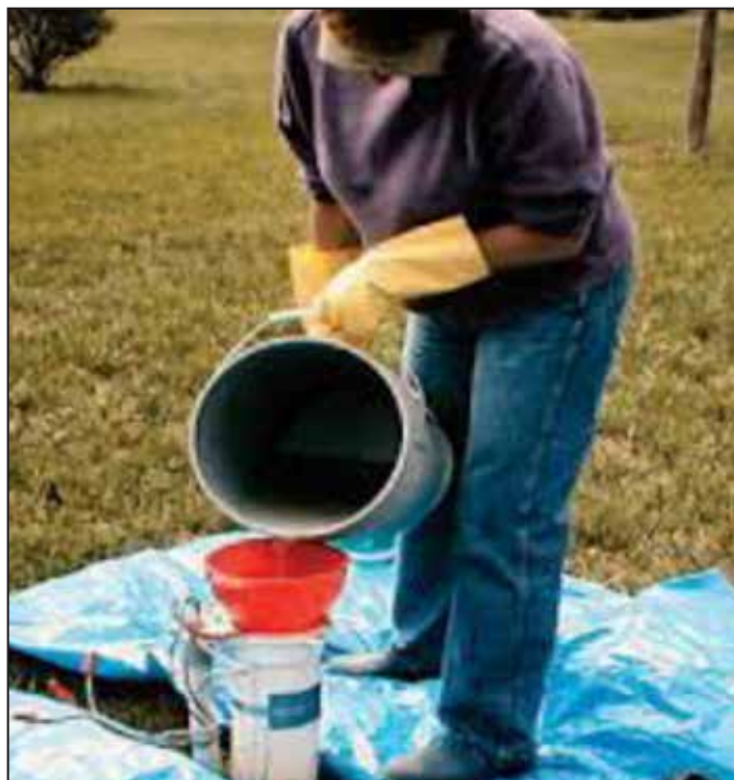
Figure 1. Shock chlorination is an inexpensive way to disinfect a well using a chlorine solution made from household bleach. (Photo courtesy of Virginia Tech University Cooperative Extension Service.)
