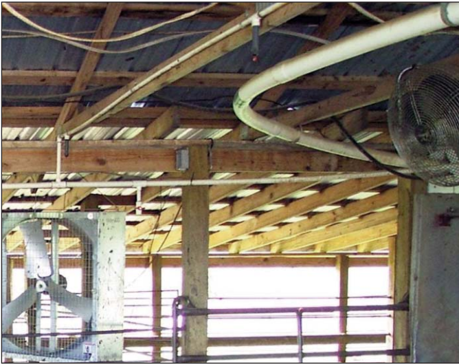
Figure 4. When hanging sprinklers, consider electrical wiring, rafters and other items affected by the sprinklers. Sprinklers that face up will not drain water when they are not under pressure from the pump unless the slope is great enough to allow the end sprinklers to be lower than the initial sprinklers.
