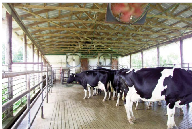
Figure 3. If fans and water run continuously, then the water droplets must be large enough so that they do not blow out of the holding pen. In addition, the manure collection and storage system should be designed to handle any extra water.
