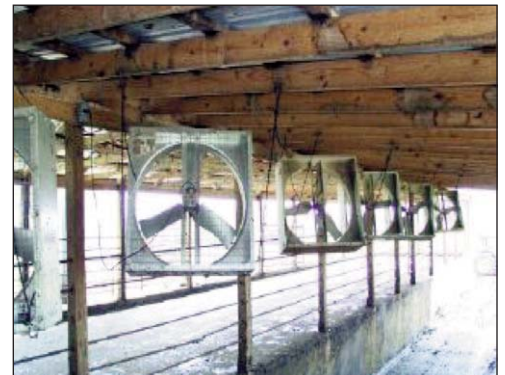
Figure 1. Used chicken house fans can be used in the holding pen, but they should have guards or be positioned where the cows and humans can't reach them.
