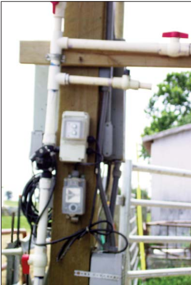
Figure 6. Adequate controls to regulate the amount of water are essential, both to conserve usage and to get the proper amount on the cows. An outlet to drain the pipes before winter and a valve to turn the water on and off are also required.
