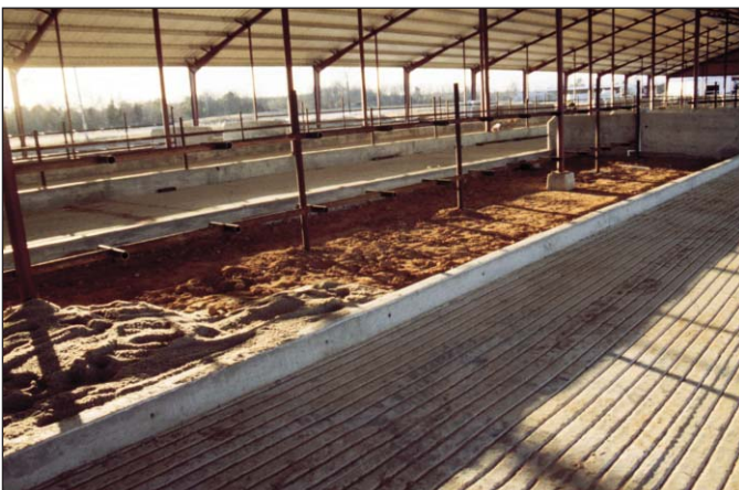
Figure 5. Concrete in the holding pen with sprinklers should be rough or grooved so the cattle do not slip. The concrete also should be well-drained so the cattle do not stand in water.
