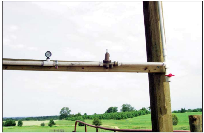
Figure 8. A pressure gauge and regulator can be beneficial in controlling variations in pressure from water systems.
