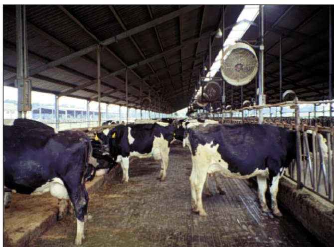
Figure 2. Fans and sprinklers in the holding pen should use the same principles as fans and sprinklers on a feeding floor.
