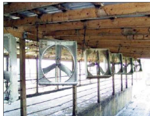
Figure 1. Used chicken house fans can be used in the holding pen, but they should have guards or be positioned where the cows and humans can't reach them.
