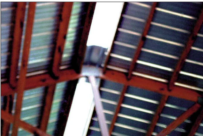
Figure 7. An open ridge row at the top of the holding pen allows heat and humidity to move away from the cows.
