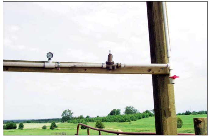
Figure 8. A pressure gauge and regulator can be beneficial in controlling variations in pressure from water systems.
