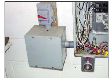
Figure 10. A percentage timer can control the amount of time for water and fans to run.
