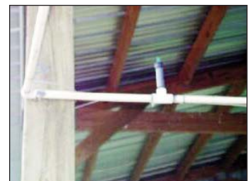
Figure 9. Sprinklers that point up maintain pressure and fill more quickly than sprinklers pointed down.
