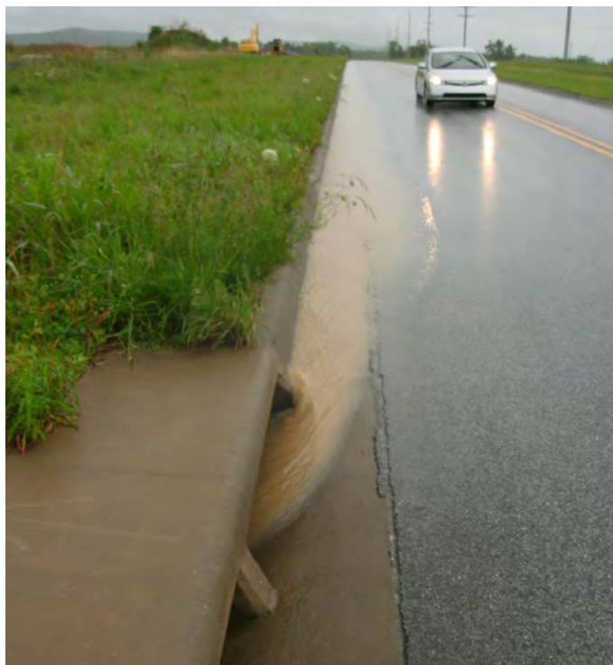
Fig. 25. Sediment carried into a storm drain that leads directly to a stream (Image courtesy of Katie Teague, University of Arkansas System Division of Agriculture)
