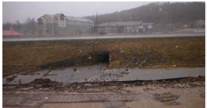
Fig. 30. Silt fence and rock wingdam BMP combination by Arkansas Highway and Transportation Department
