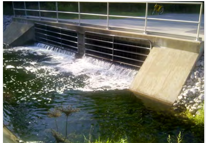
Fig. 23. Point source discharge from a municipal wastewater treatment facility (Image courtesy of CH2M Hill)
