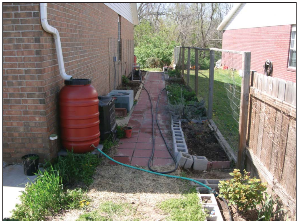
Rain barrel with soaker hose attachment leading to a flower bed
