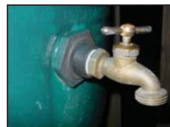
Spigot attached to a bulkhead tank fitting
