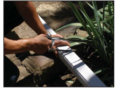
Making the gutter cut for new elbow placement
