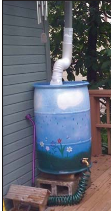
Painted rain barrel on stand with flexspout attachment
