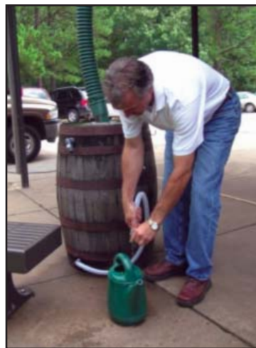
Rain barrel placed without a stand will have reduced water pressure
