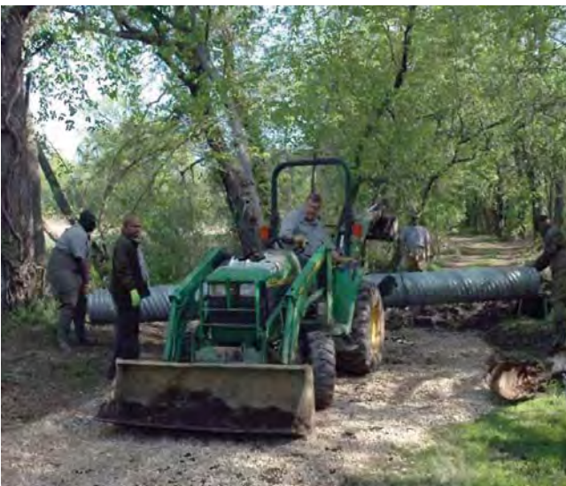
FIGURE 22. Install a culvert pipe which can handle high water and is flush with the stream bottom with rocks around the upstream end to reduce erosion. Photo by Doug Rowley, National Park Service.
