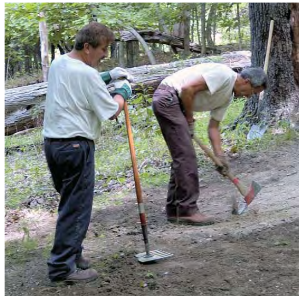
FIGURE 1. Hand tools such as a Pulaski (right) and McLeod fire tool (left) can be used to construct and maintain trails. Photo by Ted Toth, National Park Service volunteer.
