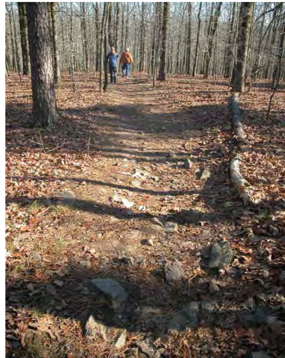
FIGURE 3. This cup-shaped trail forces water down its center and is not sustainable. Rocks, side logs and other debris that funnel water onto the trail should be removed periodically. Photo by Becky McPeake, UA Division of Agriculture, Cooperative Extension Service.
