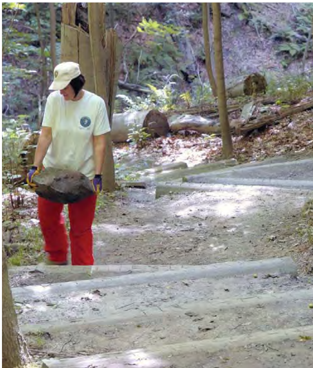
FIGURE 19. A climbing causeway gradually builds the tread grade in sections. Photo by Ted Toth, National Park Service volunteer.
