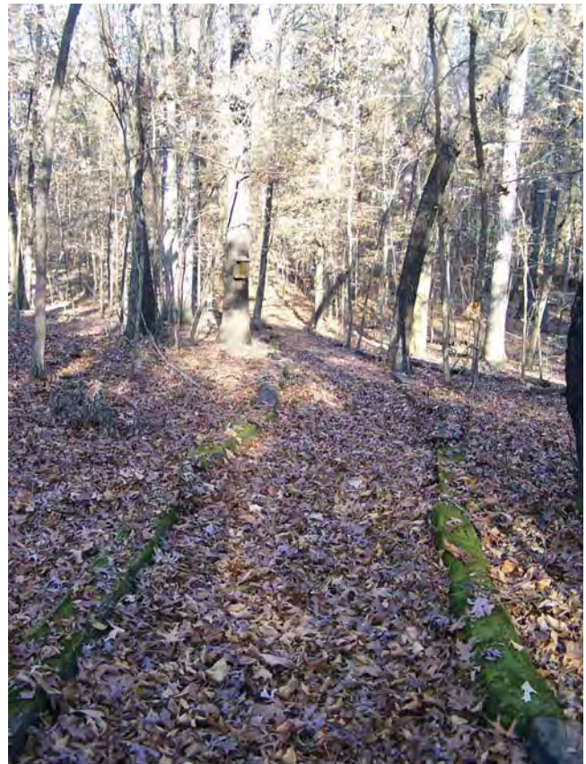
FIGURE 13. Do not edge your trail with logs or rocks as these funnel water down your trail causing erosion. Leaves are poor tread because they do not compact well, can become slick and are easily displaced. Photo by Jamie Schuler, University of Arkansas at Monticello.
