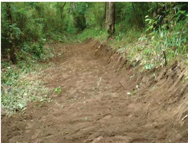
FIGURE 4. A sustainable trail with soil tread having a 4- to 6-percent outslope (1.5 to 3 inches from high side to low side). Photo by Glen Moody, National Park Service, Buffalo National River.
