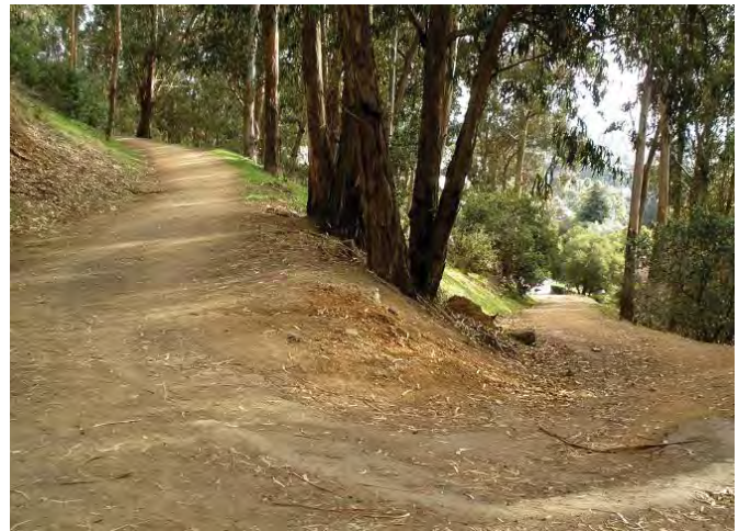
FIGURE 18. Switchbacks help the user traverse a steep slope at a comfortable pace. Photo by Ken Cheetham.
