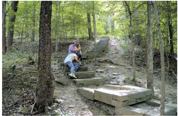
FIGURE 20. Box steps aid hikers with navigating steep slopes. Photo by Ted Toth, National Park Service volunteer.
