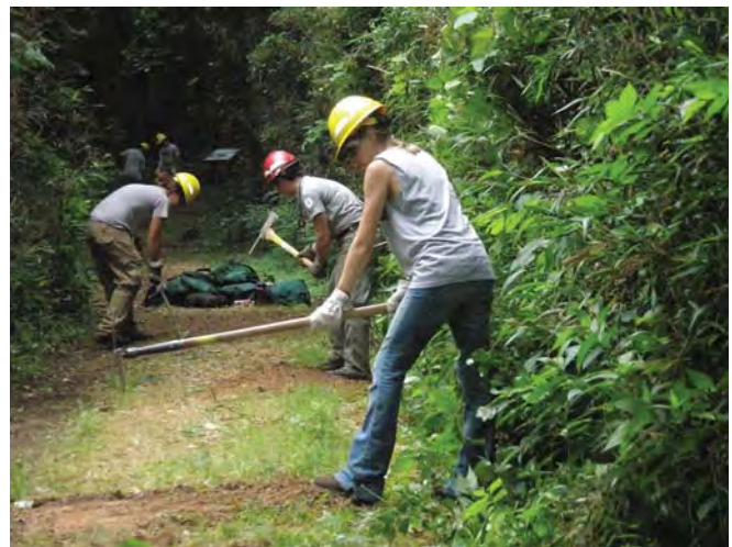
FIGURE 26. Trails may require periodic maintenance to fix problems with slough and berm. Photo courtesy of the National Park Service.
