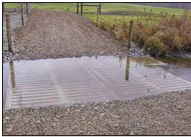
FIGURE 7. Example of a well-constructed cattle crossing. These structures help maintain streambank stability by allowing cattle to cross the water at certain locations only. Stream crossings vary in design and costs. Photograph courtesy of NRCS.
