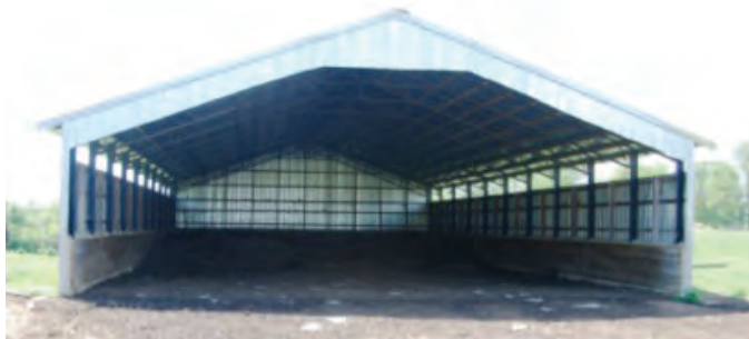
Poultry litter stacking sheds provide safe, temporary on-site storage of litter by keeping the litter dry and contained. (Photo courtesy of Rich Mountain Conservation District)
