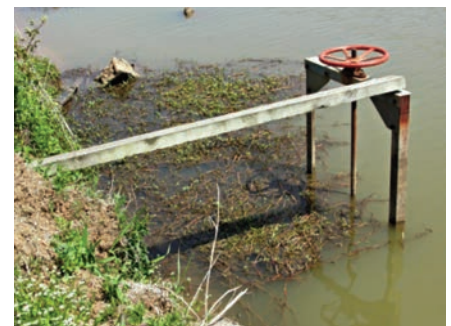
Figure 7. Water control structures are tools for providing shorebird habitat in impoundments. Image courtesy of Becky McPeake, University of Arkansas.
