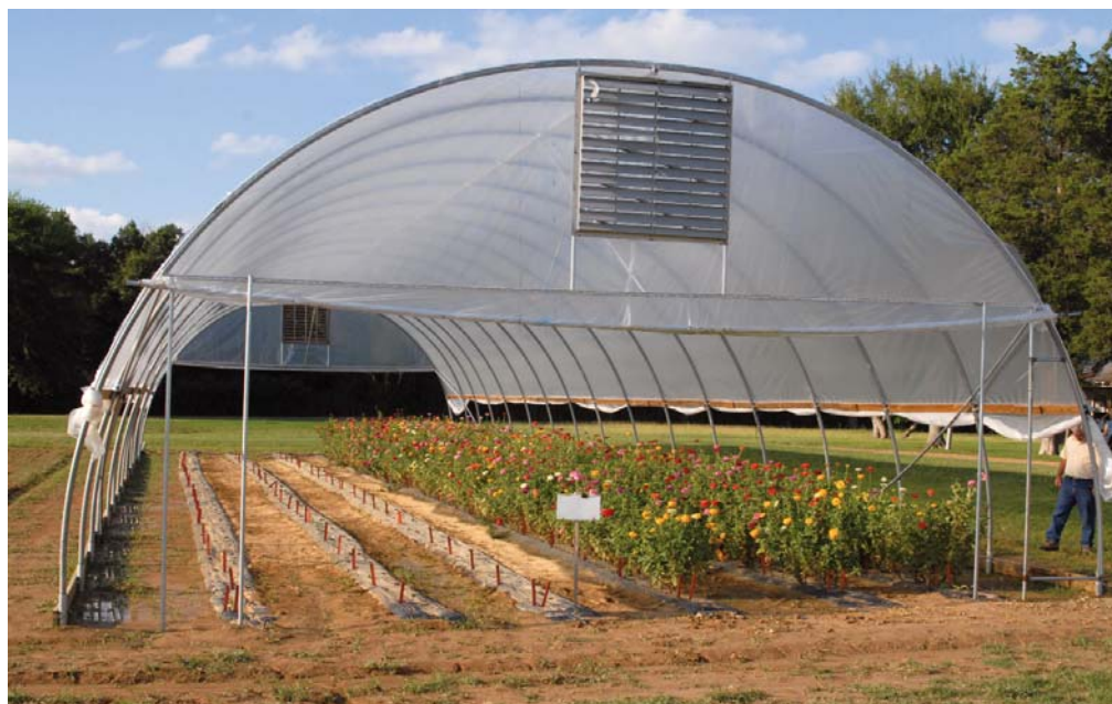
FIG. 1. Typical Quonset-style high tunnel design
