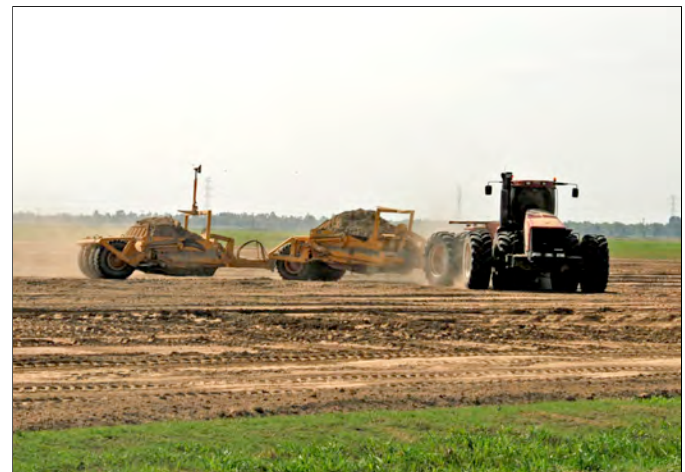
Figure 2. Land leveling to ensure good drainage.
