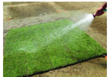
Figure 6. Begin to water the lawn thoroughly after the sod is installed and rolled.
