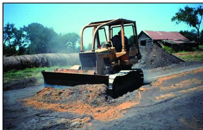
Mixing of fly ash and clean clay soil.
