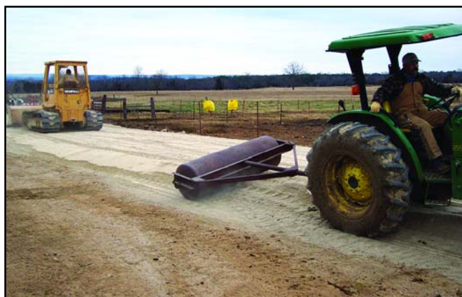
Blend of bottom ash and fly ash being spread and packed.
