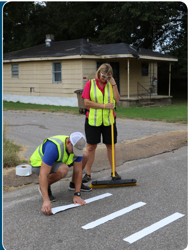
ArDROP team members put down a temporary crosswalk with pavement grade reflective tape in Forrest City, Arkansas. Photo credit: Caitlin Palenske
