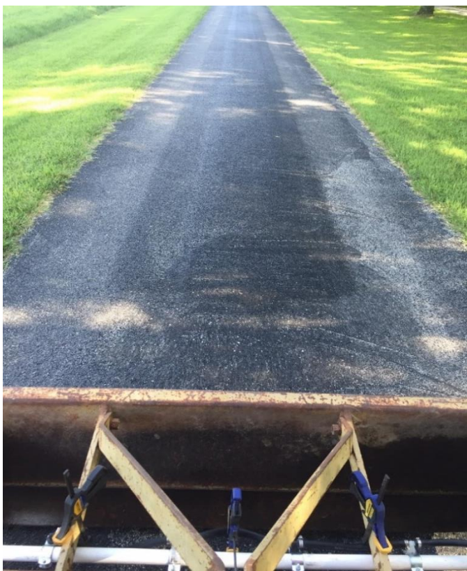
Below: Testing on driveway to insure uniform coverage
