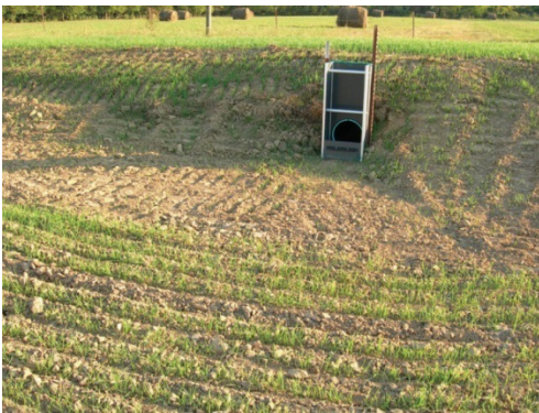
Figure 38. Water control structures allow manipulation of the water level in ponds and areas flooded for wildlife using a dike or levee.
