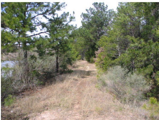
Figure 28. This fish pond dam will likely have problems with leakage (if not already) and breakage if the trees are not killed or removed.
