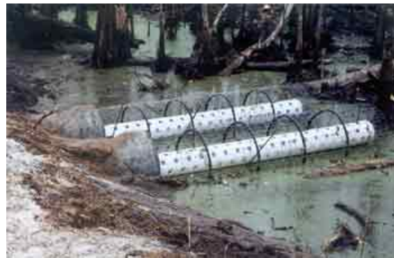
Figure 39. These two Clemson Beaver Pond Levelers were installed by the U.S. Forest Service to improve water flow through culverts and avoid beavers plugging them.
