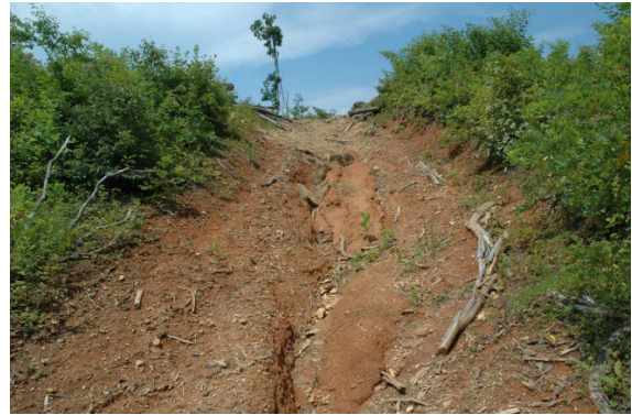
Figure 12. Forest roads should not be constructed perpendicular to slope. Roads such as this should be closed and planted to trees or shrubs.
