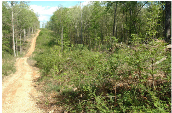
Figure 14. This forest road was daylighted to provide additional browse, soft mast, and nesting cover for various wildlife species. The road was graveled to prevent erosion because it receives considerable traffic from land managers.
