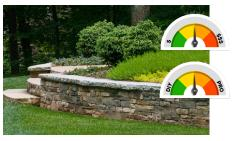
TERRACED LANDSCAPE Sloped landscapes create the potential for erosion. Terracing the slope by creating a structural wall on the downslope face can slowdown excess runoff. Planters can be used for added green space.
