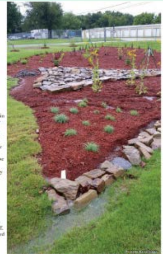
Bioswales such as this one in Springdale are very effective at controlling and cleaning stormwater runoff from the many roads and pavements in our urban environment.
