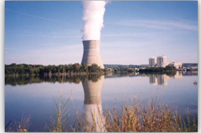
Industrial Water Supply
