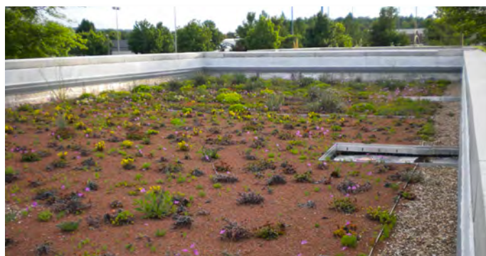
Fig. 49. Green roofs like this one at the University of Arkansas in Fayetteville can help reduce stormwater runoff (Image courtesy of University of Arkansas System Division of Agriculture)
