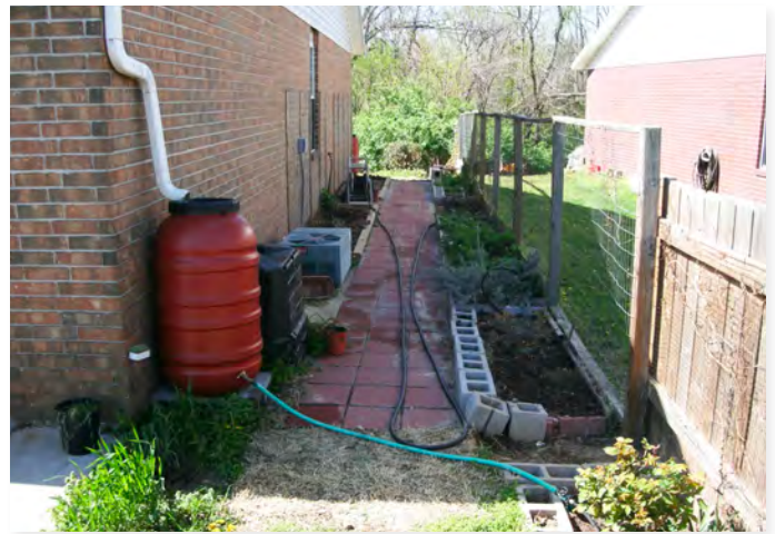
Fig. 56. Rain barrels can harvest rain water and help prevent rooftop runoff from flooding neighbors or encountering pollutants on its way to a stream (Image courtesy of University of Arkansas Division of Agriculture)
