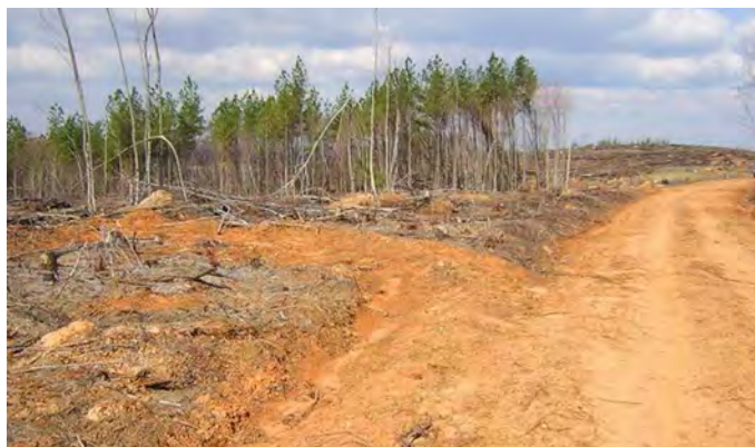
Fig. 54. Wing ditches are common forestry BMPs used along dirt roads (Image courtesy of Hal Liechty, University of Arkansas at Monticello)
