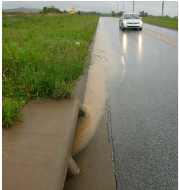
Fig. 25. Sediment carried into a storm drain that leads directly to a stream (Image courtesy of Katie Teague, University of Arkansas System Division of Agriculture)
