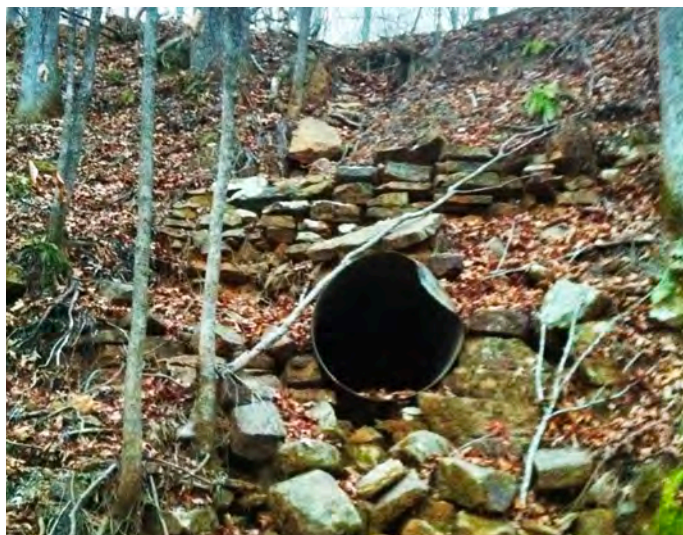
Fig. 55. Culverts and cross drains allow water to move off of forest roads into existing vegetation or downslope ditches to prevent soil erosion (Image courtesy of University of Arkansas at Monticello Forest Resources Center)
