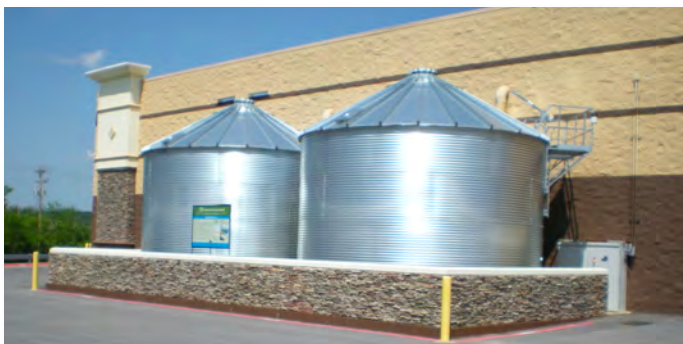
Fig. 46. Cisterns can be used to capture rooftop runoff for later reuse (Image courtesy of University of Arkansas System Division of Agriculture)
