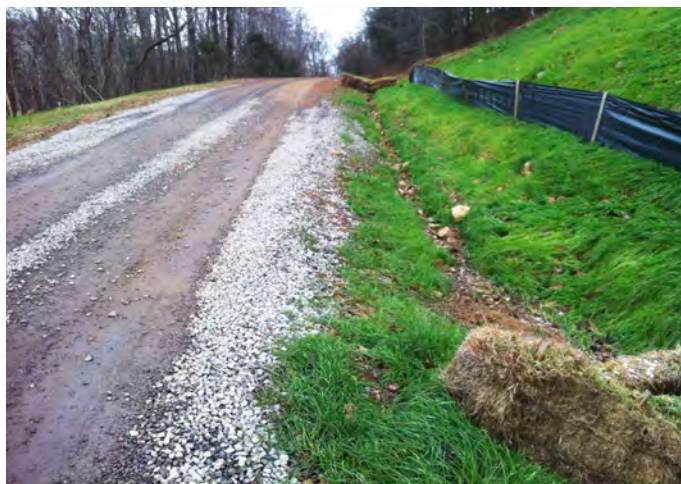
Fig. 53. Revegetation after forest road construction or maintenance prevents erosion (Image courtesy of University of Arkansas at Monticello Forest Resources Center)
