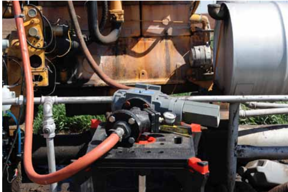
Gas meters are directional, so installation orientation is critical.
