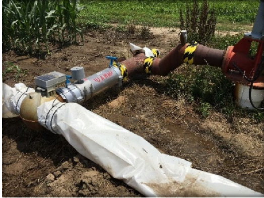
Figure 5. Example of Universal Hydrant Sealing
