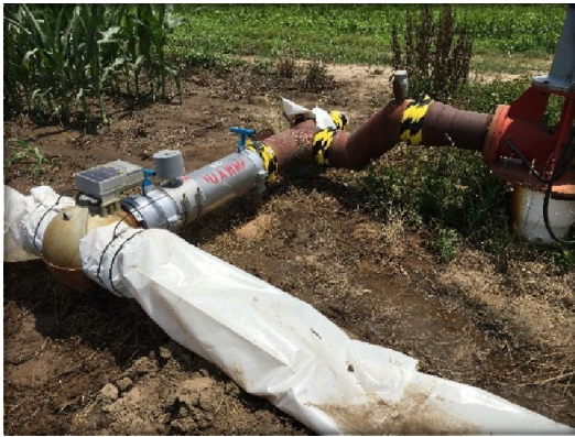
Figure 4. Example of universal hydrant sealing.
