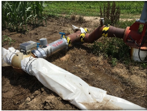
Figure 3. Example of Meter Sealing
