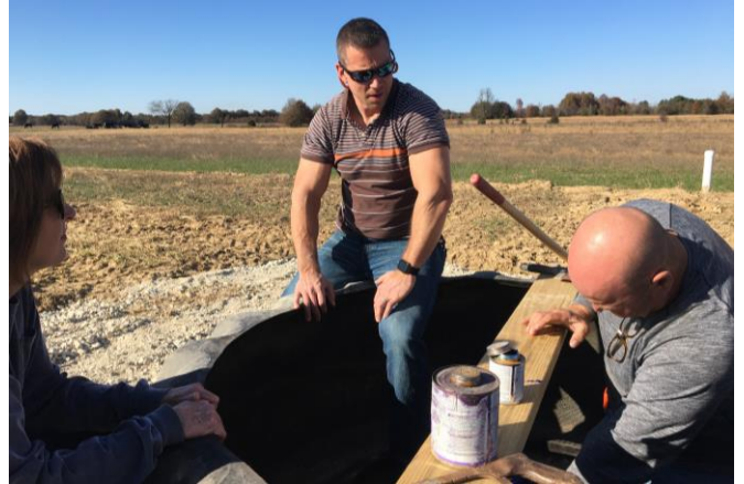
11/2020- Project team & producers work to build tire water tanks.
