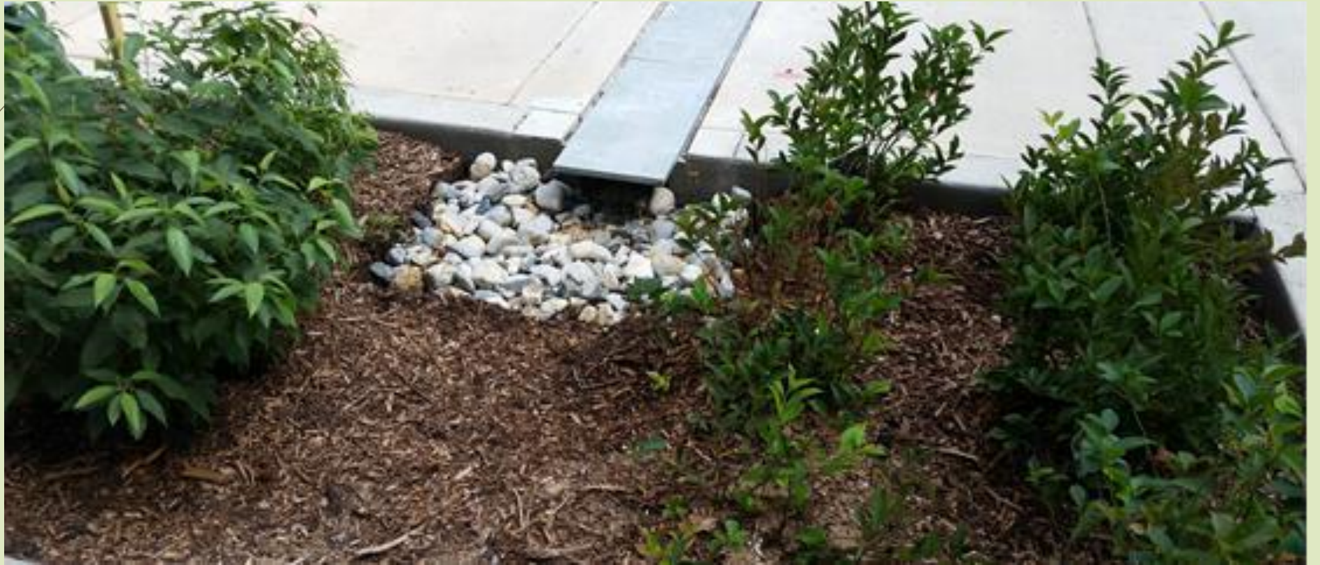
Raingarden with Run-off Scour Prevention Area
