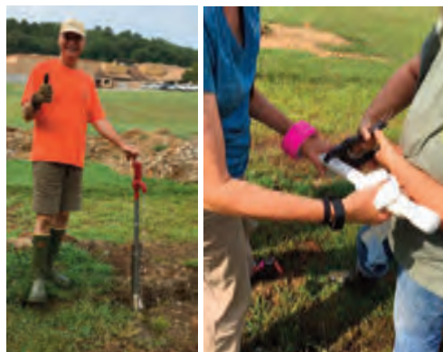
Digging trenches and cutting pipe.
