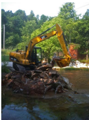
The low water bridge on Hamestring Creek in Fayetteville, Ark., the cause of erosion that threatened Gardie Dalton's house, is removed, thanks to donated equipment and service from the Rogers Quarry Group and Riggs Caterpillar of Springdale.
