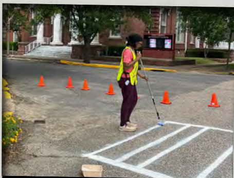
The Arkansas High Obesity Program recently helped establish two new crosswalks in downtown Marianna at the intersections of Poplar and Main streets and Poplar and Mississippi streets.
